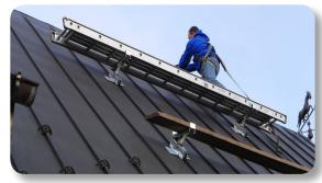
roofer's belt. Installing a SeamSAFE anchor takes a minute or less and only requires a single wrench to tighten three bolts.
