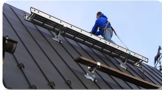
roofer's belt. Installing a SeamSAFE anchor takes a minute or less and only requires a single wrench to tighten three bolts.
