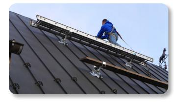
Complete Safety System: SeamSAFE anchors can be used along with SeamSAFE roof brackets to provide the ultimate fall-arrest system. Together, they offer secure support for standing seam roofers, their tools and roofing materials.
